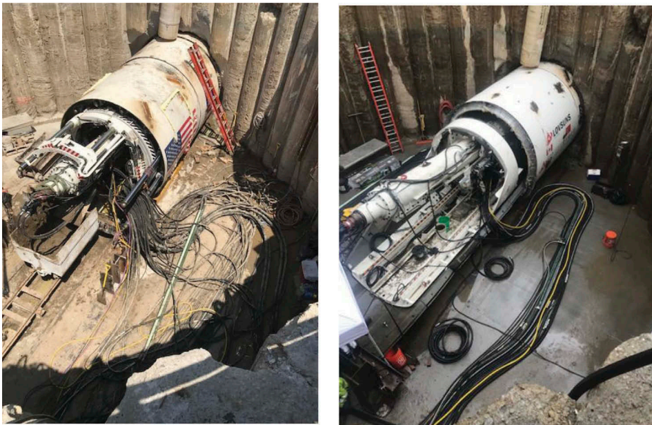
Figure 4. Launching the TBM (left) and half-ring installation for TBM propulsion (right).
