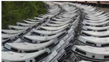
Image 6: On-site storage of BarChip fibre reinforced segments after transport.
