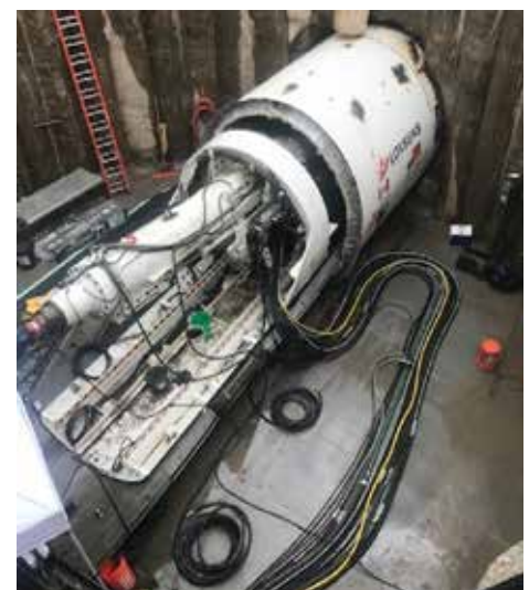
Image 3: Blacksnake TBM launch with BarChip fibre reinforced "half-ring".
