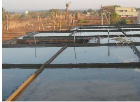
Ponding method of concrete curing.
