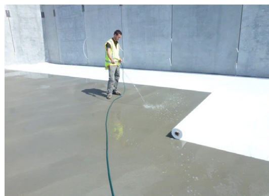
Plastic film for concrete curing.
