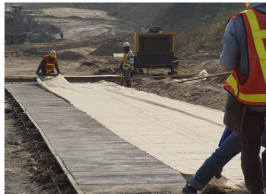
Burlap material for concrete curing.
