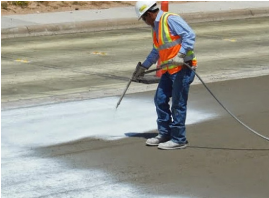
Application of curing compounds.
