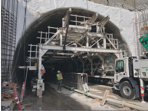
Figure 5. Tunnel Rebar Gantry in Place at the Face of the South Portal Tunnel Entrance
