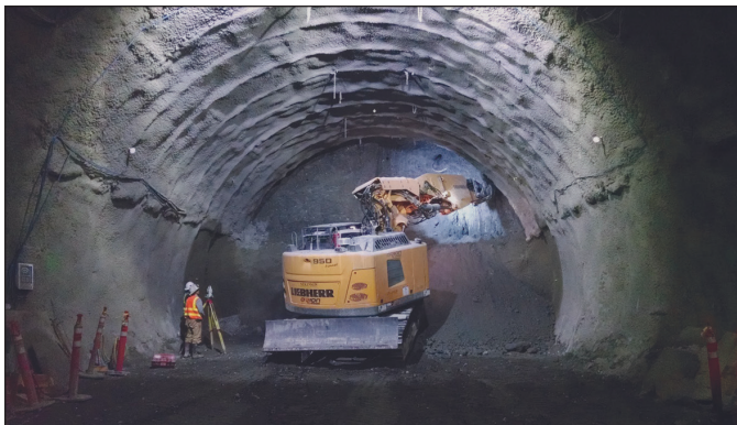
Figure 2. Three-Heading SEM Tunnel Excavation
