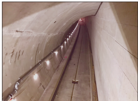
Figure 7. Use of Shotcrete as the Final Lining in the Expanded Zone and in the Tunnel Center Wall
