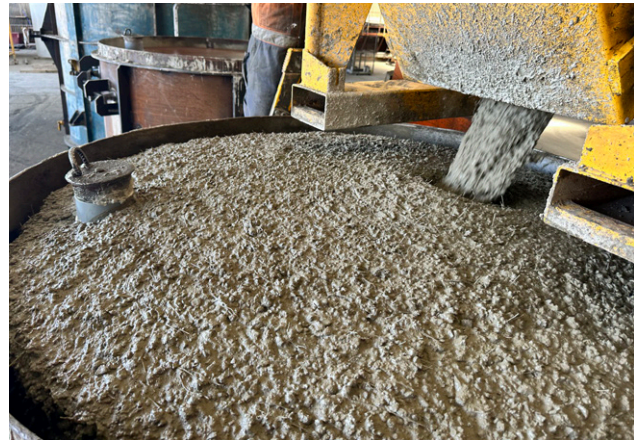
Casting Septic Tanks
