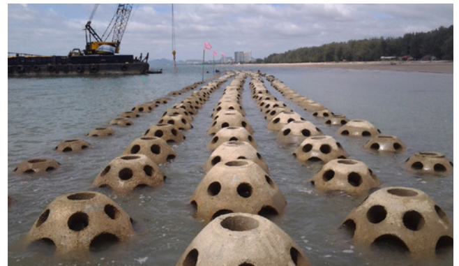
Erosion Control Dome Barriers: Enabled removal of concrete cover, reducing thickness from 150 mm to 50 mm.
