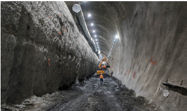
Melbourne Metro: Eliminated the need for 50 mm smoothing layer, reducing overall shotcrete consumption by 15%.
