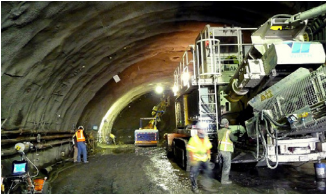
Caldecott 4 th Bore: Load Sharing Design allowed final lining thickness to be reduced by 30%
