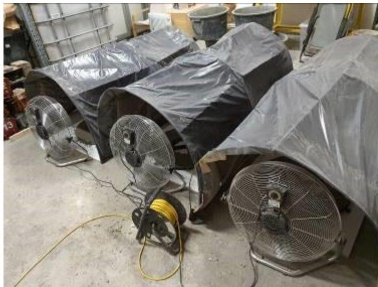
Figure 8. Installation of the moulds and the fan
