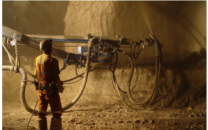
Figure 3. Spraying a fibre reinforced shotcrete tunnel lining onto hard rock to provide local support.
