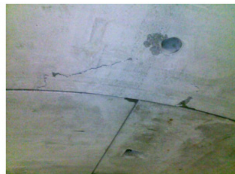
Figure 6. Cracks in fibre reinforced concrete segments. These will be subject to hoop loading while in service and could either widen or become closed depending on the magnitude of axial loads and bending moments.
