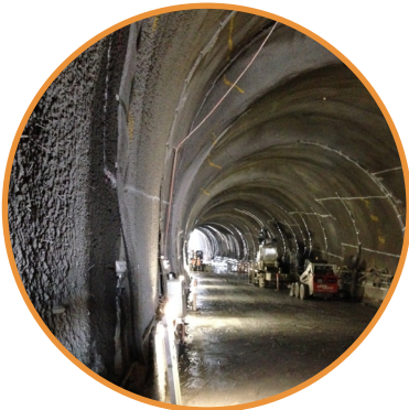
BarChip reinforced shotcrete lining.
