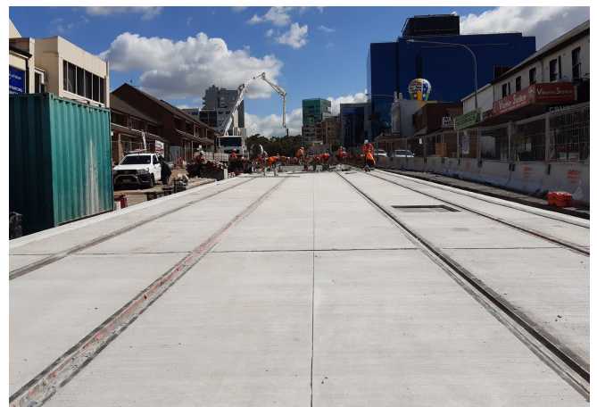
Finished Trackslab - Parramatta Light Rail
