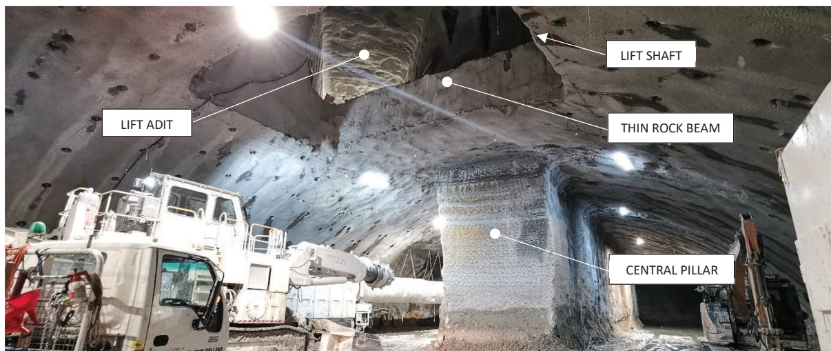
FIG 5 – Excavation of cavern central pillar under lift shaft and lift adit.
