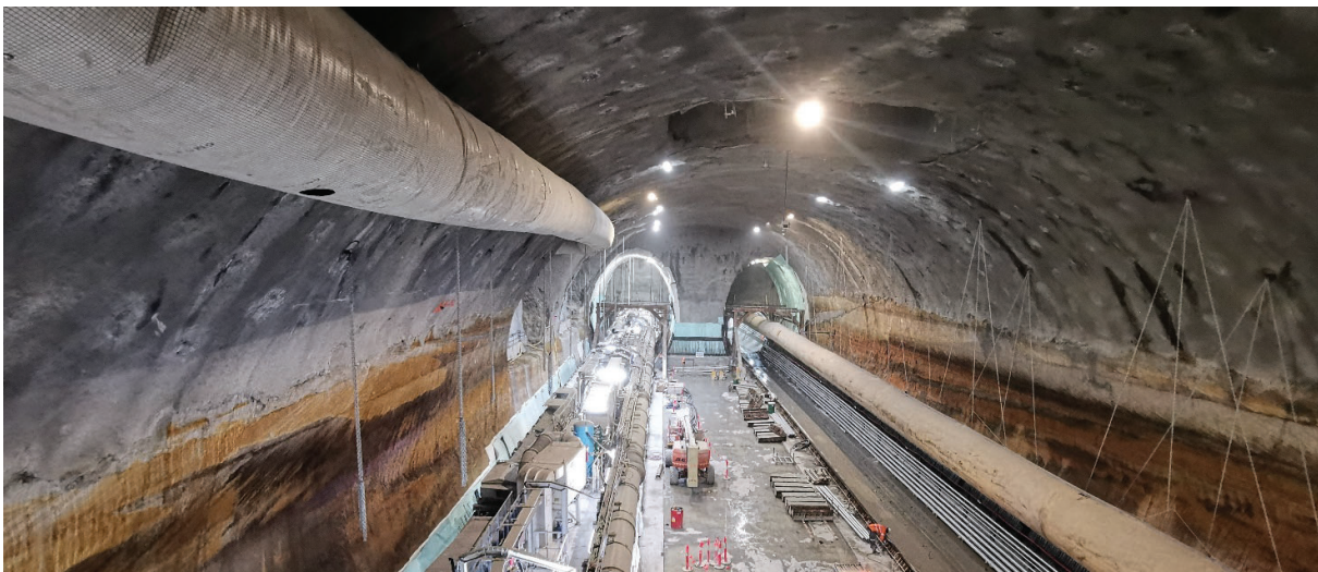
FIG 7 – TBMs traversed through completed cavern.
