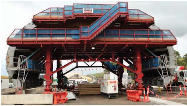
FIG 4 – Formwork shutter.
