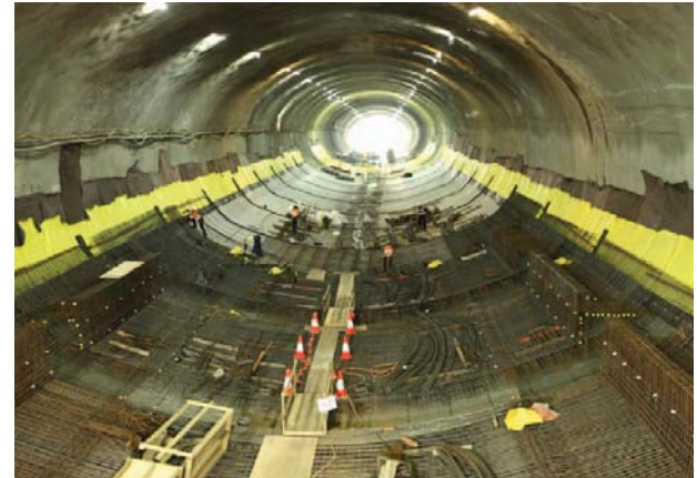
FIG 6 – Waterproofing membrane and reinforcement in the invert.
