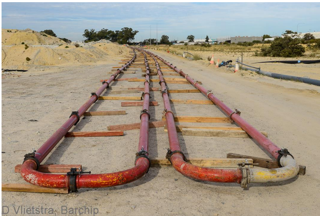
Figure 3. 1500m of pump line set up for the trial
