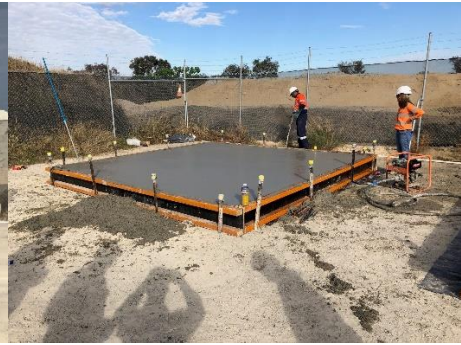
(b) Finished slab in pre-construction trials
