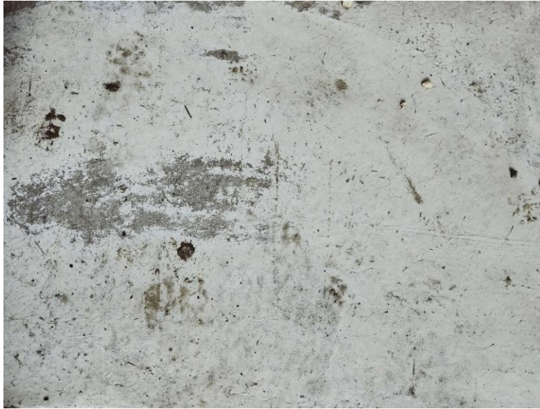
(c) MSFRC slab after 1 year
