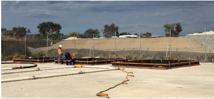
(a) Pre-construction trials
