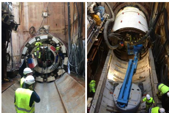
Figure 7. Preparation for the tailskin assembly (left) and complete shield assembly ready to bore (right)
