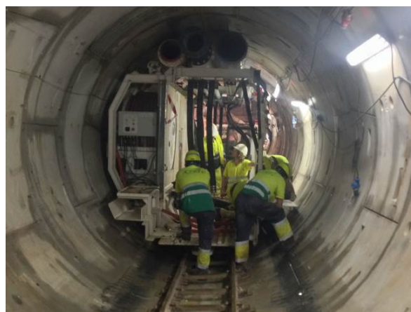
Figure 16. Pushing operation of gantry 9 towards the back-up prior to assembly it in its final position
