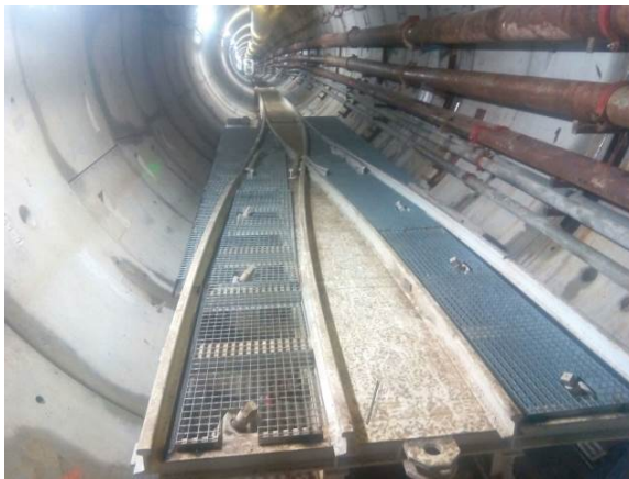
Figure 17. California rail switch installed in the tunnel
