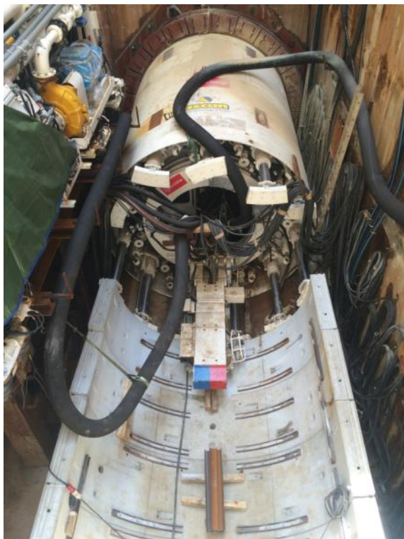
Figure 23. “Half-ring” segment structure used to push the mixshield during the start of excavation
