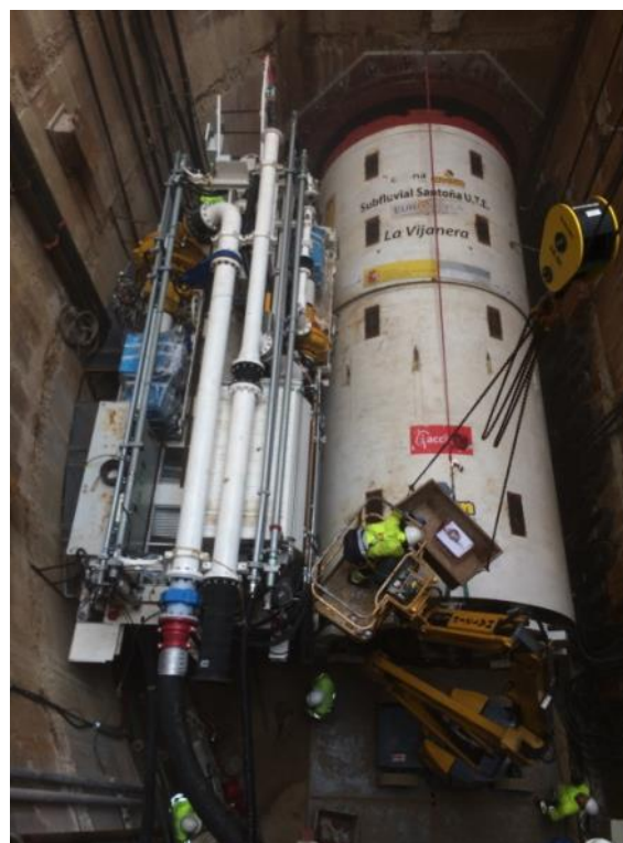
Figure 5. Assembly of the shield, thrust pipe and gantry 1 (on top of a structure) in the bottom of the shaft
