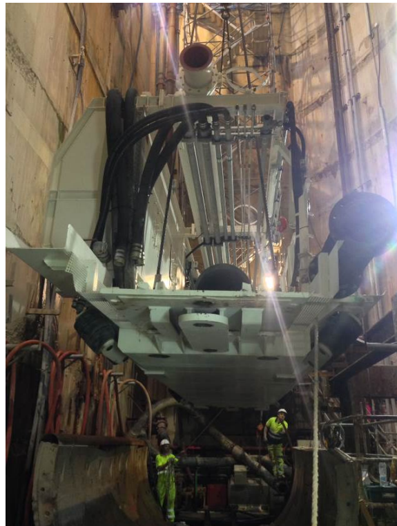
Figure 12. Lifting and positioning of gantry 4 in the bottom of the shaft
