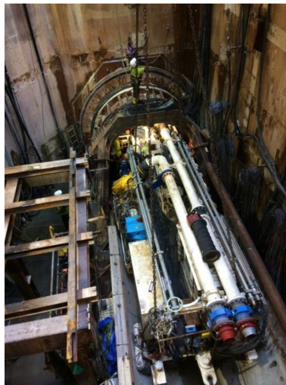
Figure 9. Lowering of the first gantry to its definitive position and services connection
