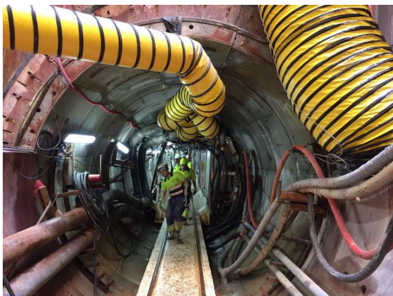
Figure 14. Disposal of temporary cables and hoses along the tunnel after positioning of gantries 5, 6 and 7.
