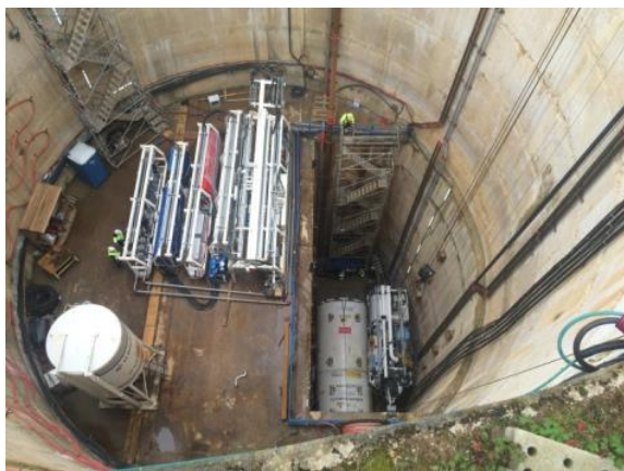
Figure 6. Assembly of the lateral parts of the gantries in the intermediate shaft floor
