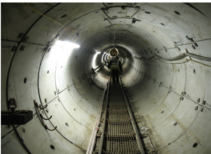
Image 4: A segmental tunnel lining is designed to be in compression, meaning isolated tensile creep of fibre reinforcement is not a factor.
