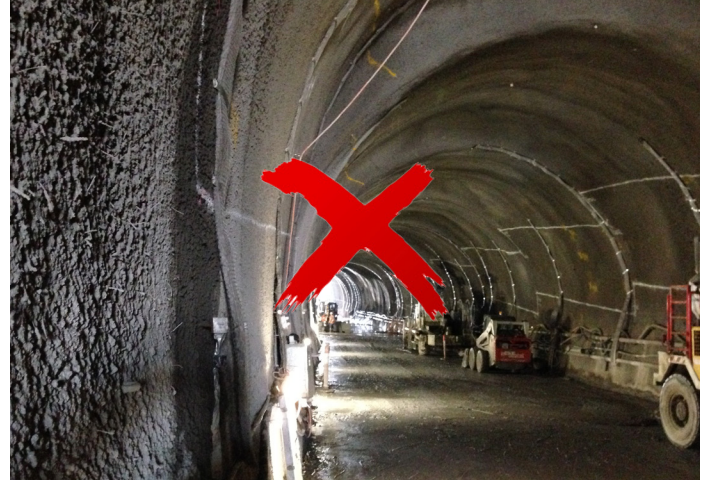
Image 1: MC2010 is not intended to be applied to slab on grade or shotcrete applications.
