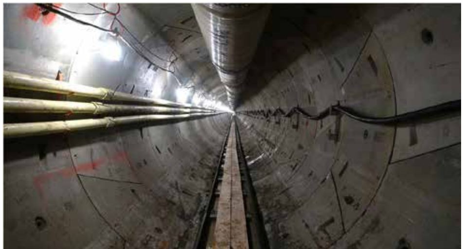
Image 7: Installed BarChip reinforced rings in the Blacksnake Tunnel.
