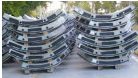
Image 5: On-site storage of BaChip fibre segments after transport.
