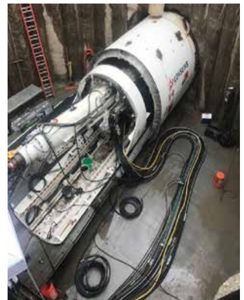
Image 2: Blacksnake TBM launch with BarChip fibre reinforced “half-ring”.
