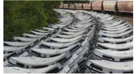
Image 4: On-site storage of BaChip fibre segments after transport.
