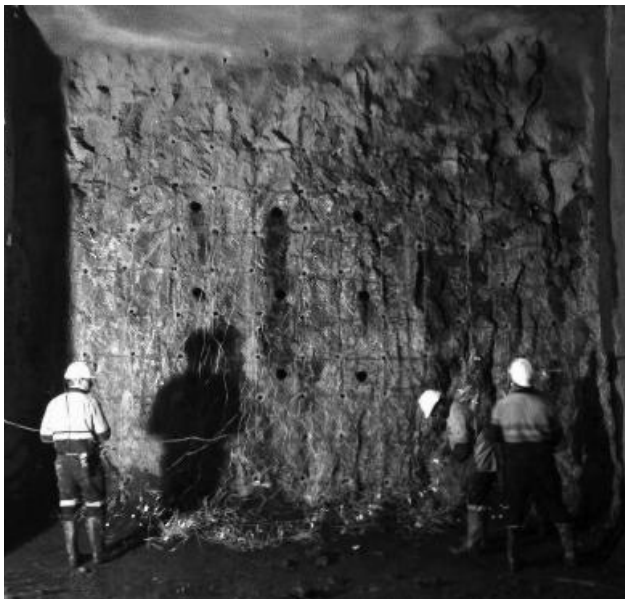
Figure 6. Cross-passages excavation in D&B.
