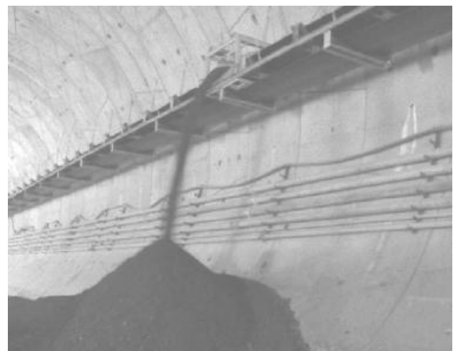
Figure 8. Discharge material along the tunnel.
