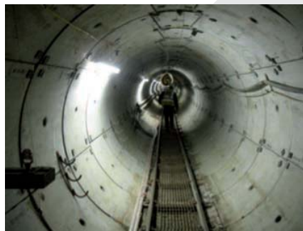
Figure 29 : Segmental lining of macrosynthetic fibre reinforced TBM tunnel
