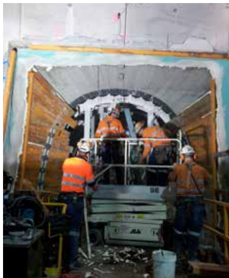
BarChip synthetic fibre reinforced cast in-situ permanent lining.
