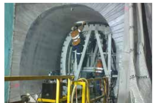
BarChip synthetic fibre reinforced cast in-situ permanent lining.
