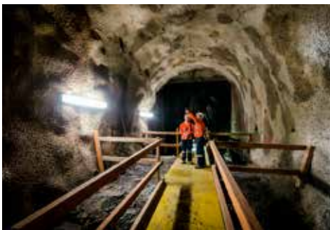
Fibre reinforced temporary shotcrete
