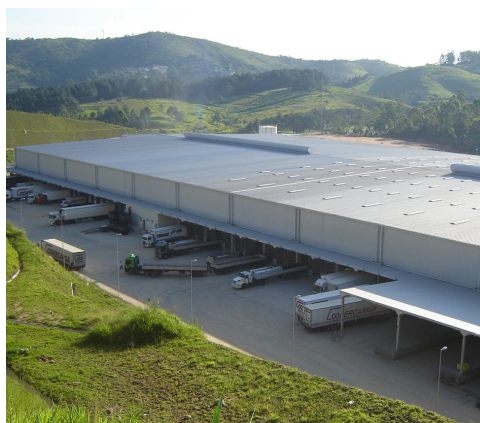
Carrefour itapevi distribution centre
