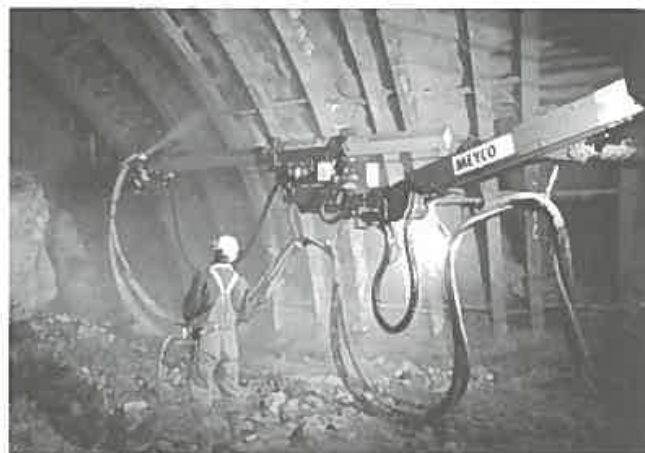
Figure 2. Wet application, robotic controlled spray rig.
