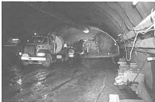
Figure 1. Example of FRS in tunneling applications.
