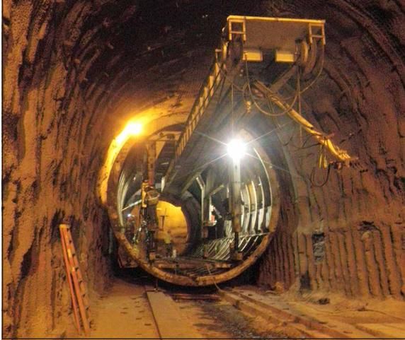
**Figure 3. Form set up for first placement**
