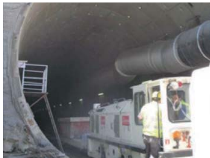
Figure 33 : Portal of the TBM tunnel
