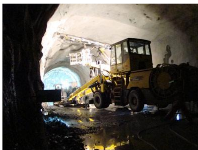
NMT excavation heading and equipment
